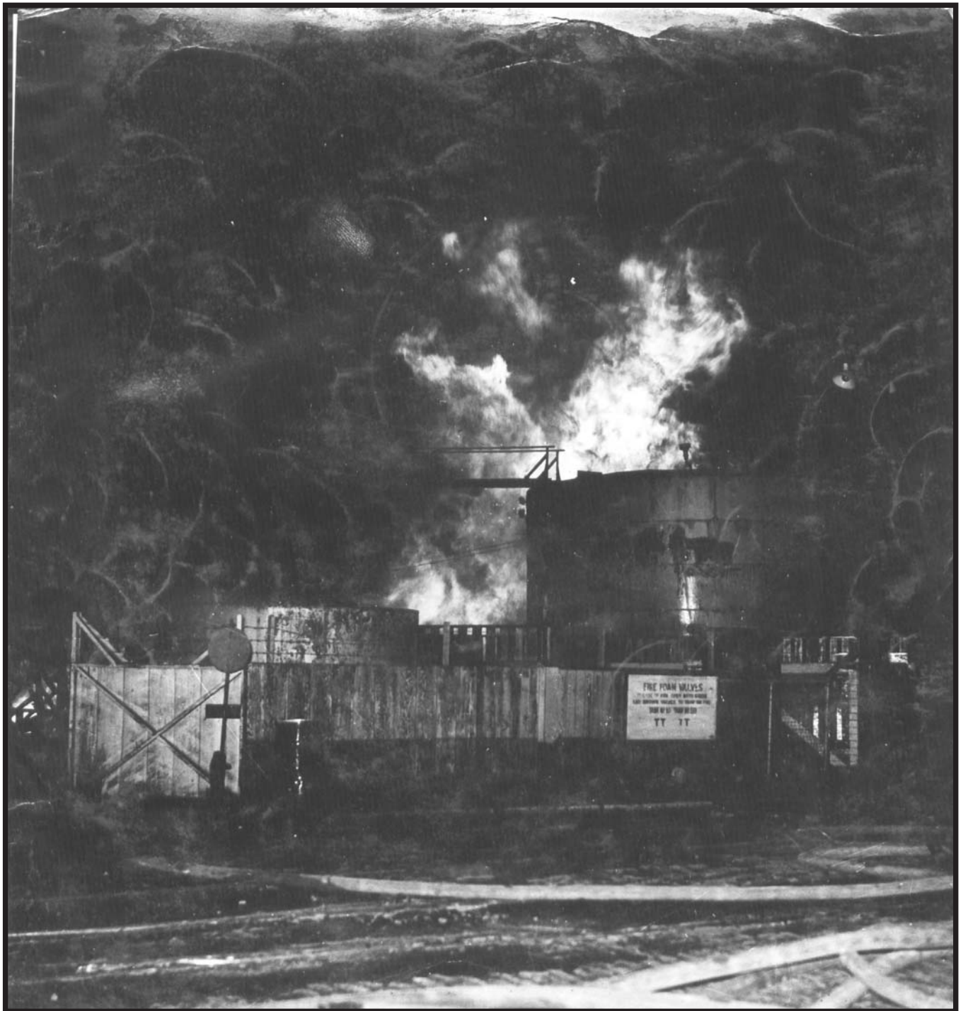
5th Alarm - September 22, 1937 07:30 hrs. 8th Street & Hooper - Standard Oil Co.
